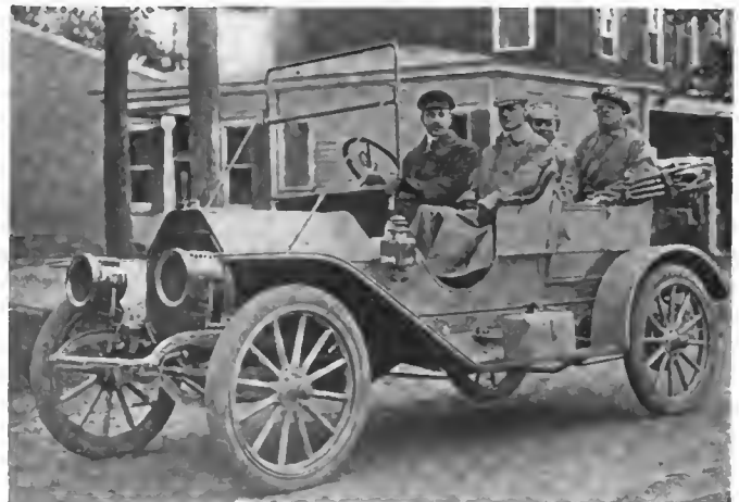
Overland "Thirty" That Carried a Notable Four
